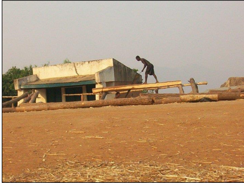
Figure 7.1: Sawyers at Likhubula cutting pine into planks for a construction project
